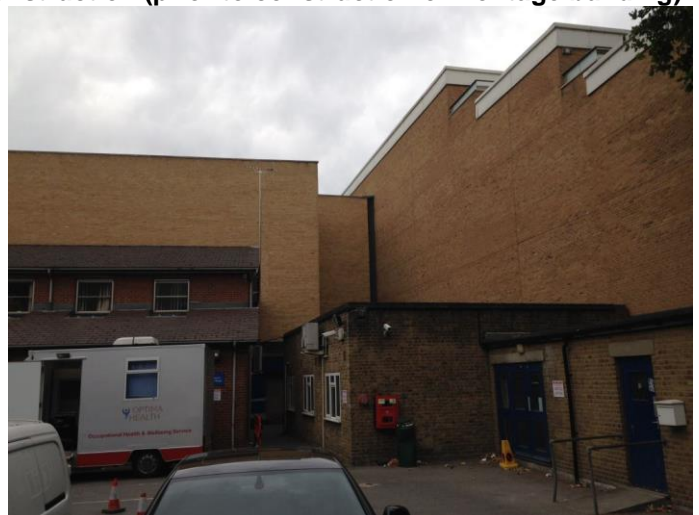
The Courtyard viewed from within the site
