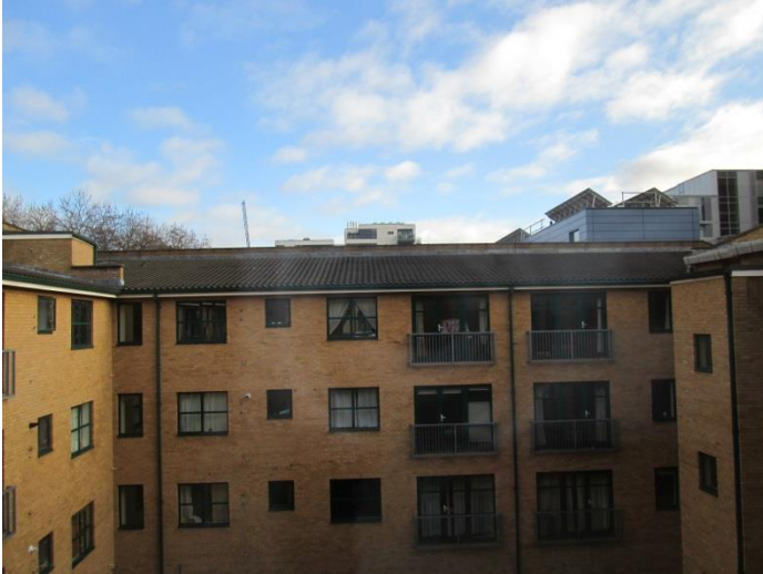
Silverdale Court internal courtyard looking east
