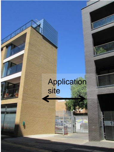
Existing entrance from Pear Tree Street
